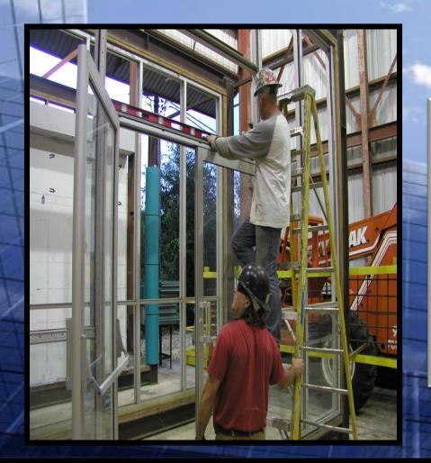
The Apprentice learns how to Install a composite panel wall, store front, curtain wall, double doors, stairs/hand rails and how to properly apply caulking and sealants.
